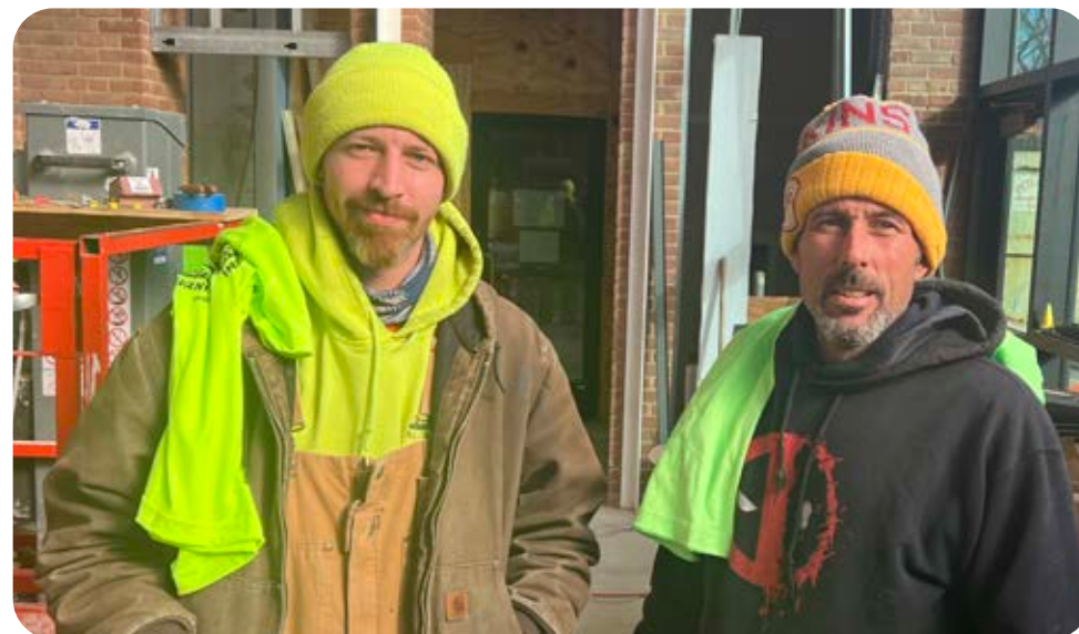
Local 181 Glazier Dave Oberacker and Local 847 Glazier Dave Gilliam working for Allied Glass at the Karamu House.
