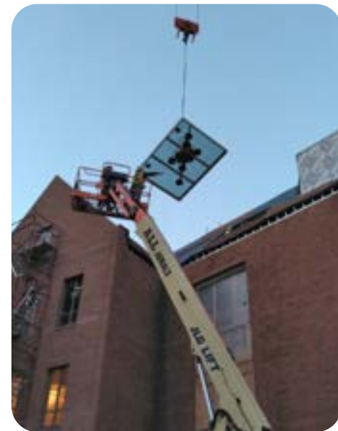
Local 1162 member Shon Neice, working for United Glass, guides the glass unit to be set.
