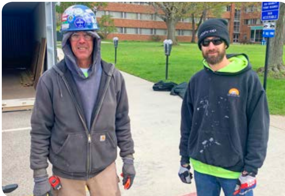
Local 181 members Dan Koontz and Tim Yurik working for RC Glass at Kent State University.
