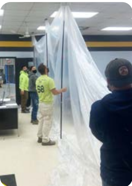
Toledo apprentices learning how to construct zipper wall.
